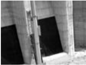
Devecikonađı HEPP Trashracks
