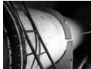
Arpa HEPP Penstock L = 870 m, \phi = 2 m
