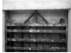
Devecikonađı HEPP Fixed-Wheel Ps = 16 m H = 5500 mm W = 4200 mm
