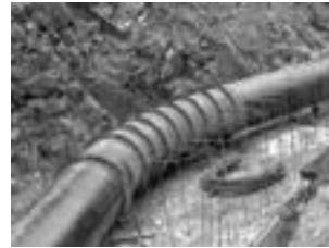
Vizara HEPP Penstock Steel, 4000 m, \phi = 1.4 m
