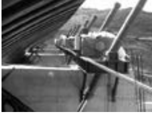
Devecikonađı HEPP Spillway Segment Gates H = 9530 mm, W = 8700 mm R = 10 m
